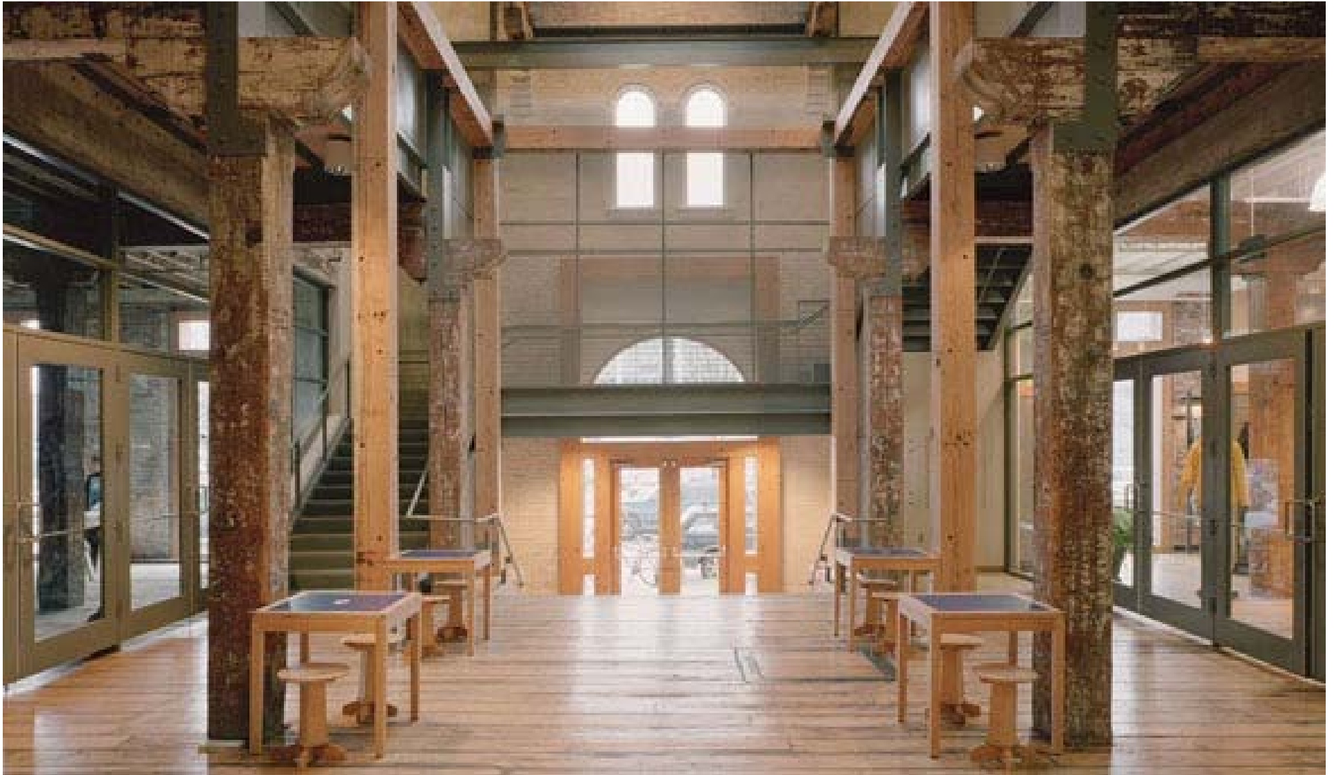
The Interior of the Ecotrust building, showing original columns unfinished and left rough, the stair (straight ahead) in light steel allowing lots of natural light.
