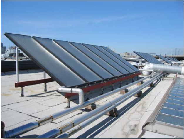
Solar panels on roof
