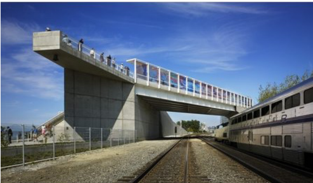
above: BNSF bridge within the park. Photo by Benjamin Benschneider
