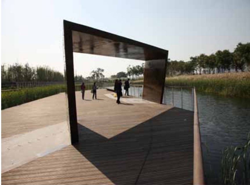
14 The steel arbor in the wetland is composed of recycled steel panels from the site, which provides shade, shelter, frames views, and shapes spaces.
