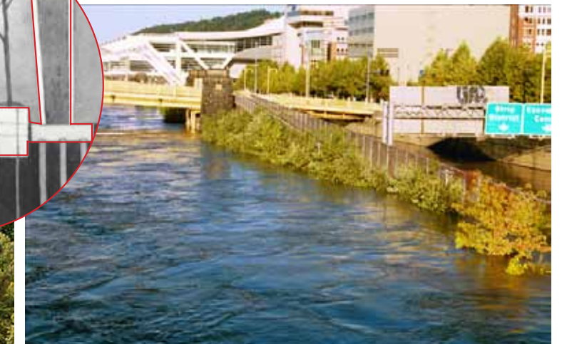
+ SEASONAL FLOODING of lower park level
