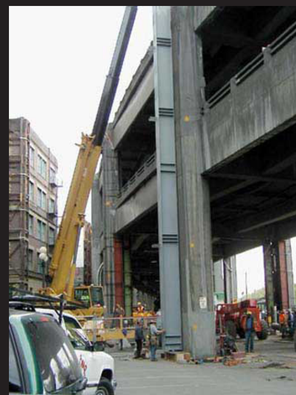
(L) Photo shows repairs by WS-DOT being completed after the 2001 Nisqually Quake. (R) The damage becomes apparent months after the quake hits when water seeps through the concrete and disrupts the structure of the Viaduct.
