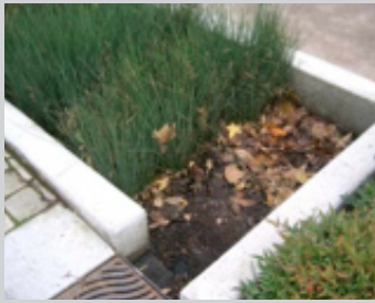
Debris build up in swale. ( http://www.portlandonline.com/shared/cfm/image.cfm?id=167503 )
