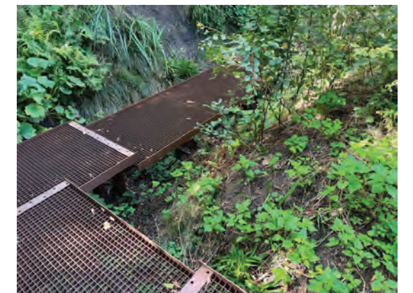
STORMWATER INFRASTRUCTURE Image Courtesy of COAST STUDIO
