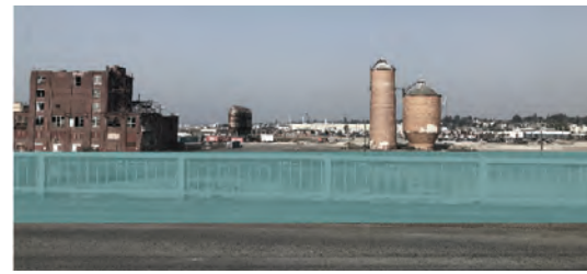
1. NO PEDESTRIAN ACCESS
