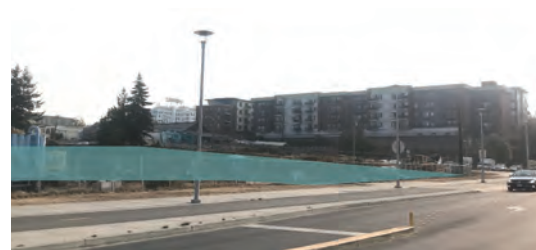
3. NO ADA ACCESS FOR SLOPE CHANGE
